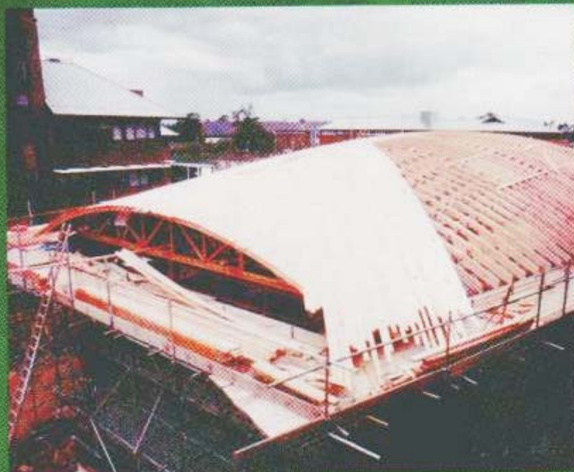
Curved trussed rafter roof at Reading University
