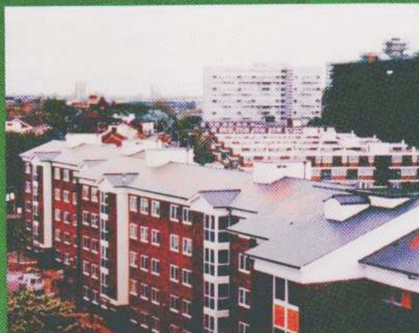
Conversion from flat roofs over social housing in London Borough of Hackney
